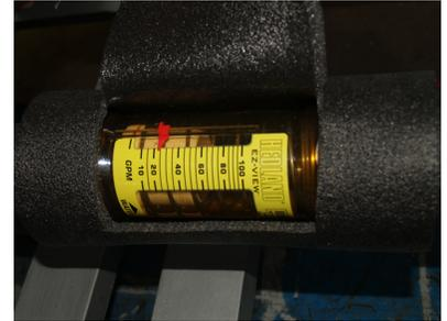
To confirm flow, check the Flow Meter. If no flow is indicated, it is likely there is an air lock in the pump and you will need to bleed the air from system. Confirm both valves are open and try cycling the power to the pump OFF and ON. If still no flow, turn power off and carefully open the plug located on the stainless steel head of the pump, bleed air from pump head and re-tighten pump head plug.
